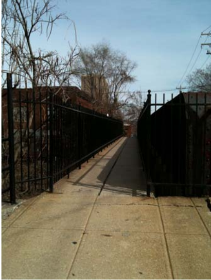
11 th Street Bridge Sidewalk Looking West
