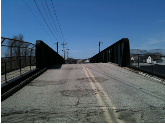
15 th Street Bridge Looking West
