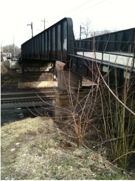
15 th Street Bridge Looking East
