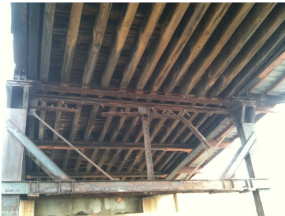
Underneath 15 th Street Bridge
