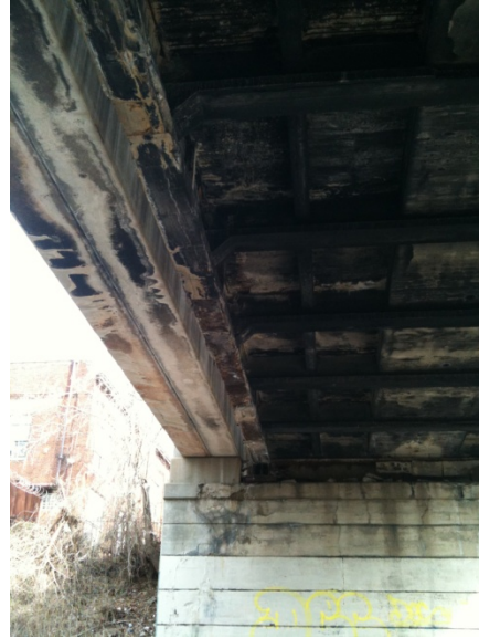
Underneath 11 th Street Bridge
