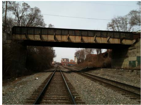
11 th Street Bridge from CSX Railroad
