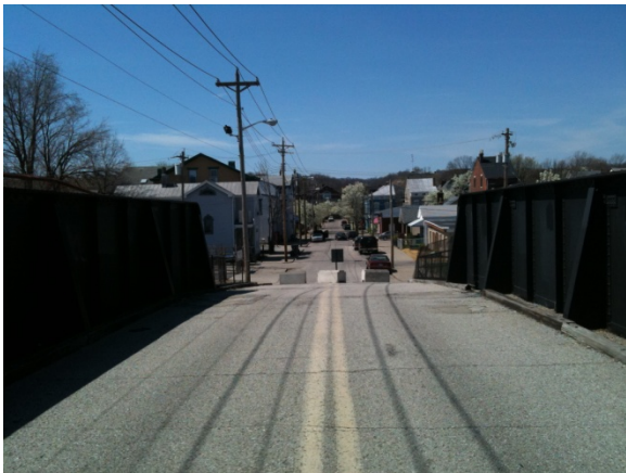
15 th Street Looking West
