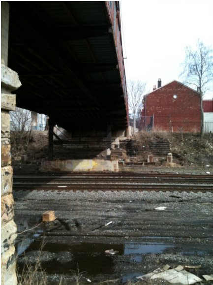
15 th Street Bridge Looking East from CSX Railroad
