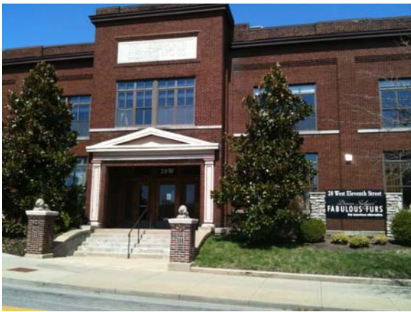
Watson Electric Company Building
