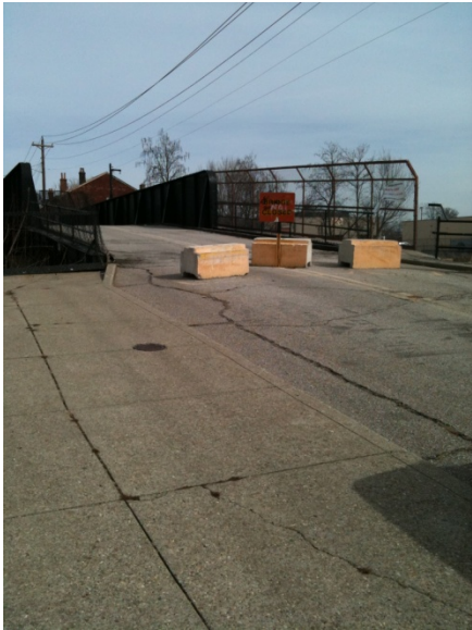
15 th Street Bridge Looking East
