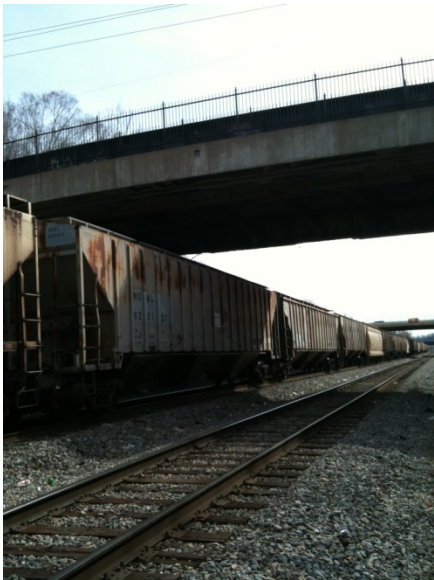
11 th Street Bridge from CSX Railroad
